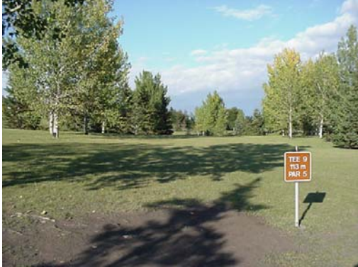
Figure 4.F, 4.G Example of Environmental Disturbance from Erosion & Mitigation Measure
